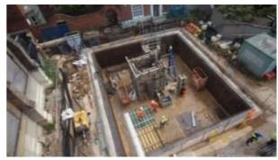
footage shows work to complete the upper basement walls, including waterproofing, insulation and concrete. The lift shaft Is clearly visible in the top centre of the site. The videos can be seen here: **Birds Eye View External**
