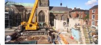
to complete the basement and then the ground-floor slab and ground-floor walls, followed by the first-floor slab.
