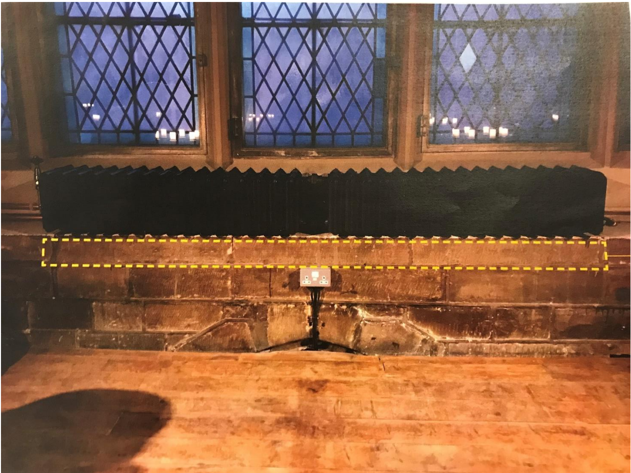
Annotated photograph showing proposed plinth location underneath the west window.
